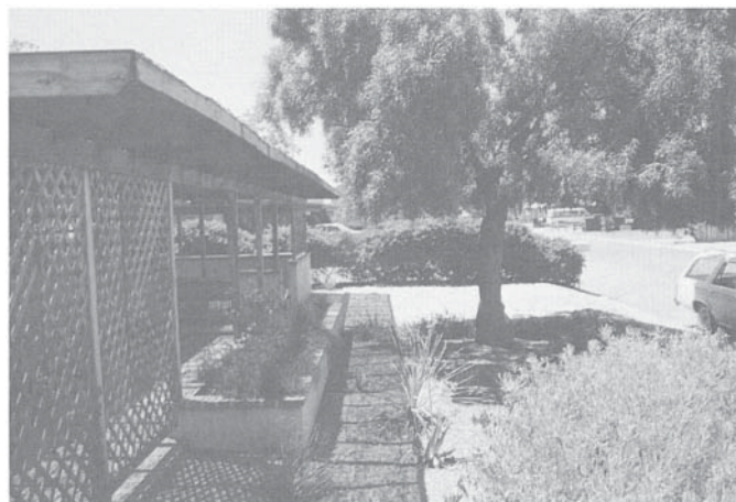
Fig. 10. Casa del Agua, Tucson, AZ. Demonstration house that meets its water needs through rainfall harvesting. Indigenous landscaping is watered by the house gray water system.
